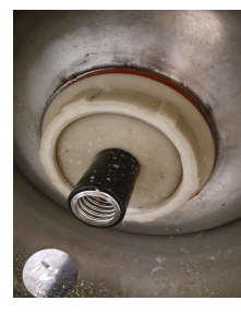
Compression Nut Inside Sump
