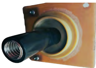
Bond to sump wall
