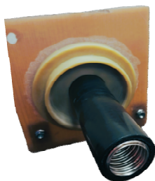
Bond to sump wall outside of the sump.
