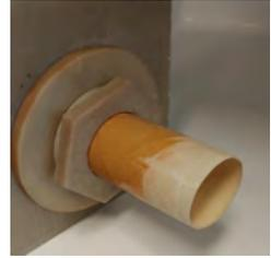
Seat the seal and thread in nut.
